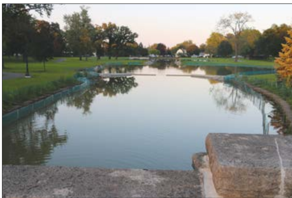
The new lagoon system at South Park was tested by recent flooding.
