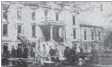
Photo from M.E. Kuehl Studio The former county courthouse demolition is shown in this 1939 photo.
