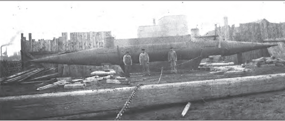
Richard Raddatz's submarine is shown being built in Oshkosh in 1897. Photo from Ed Tiedje
