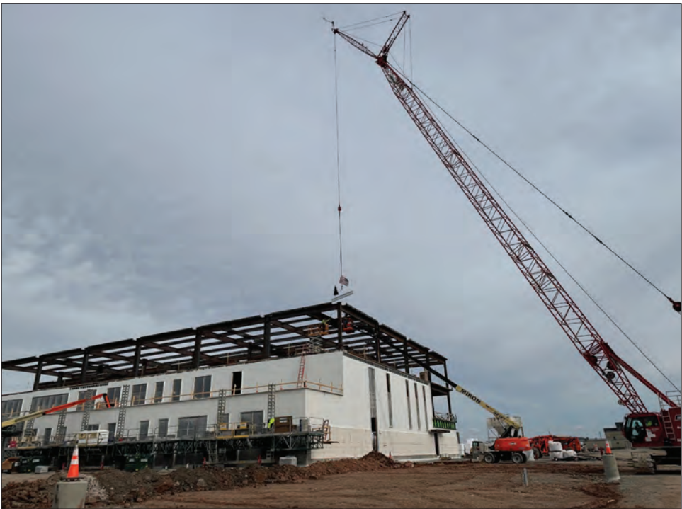
A final steel beam is added to the top of ThedaCare Medical Center-Oshkosh last Wednesday as the project progresses on 6th Avenue and Oregon Street.
